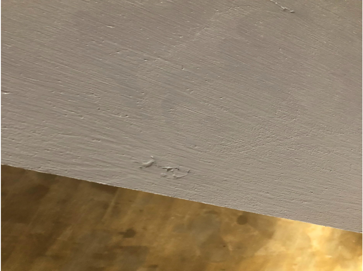
A knot/imperfection in the sheet that was filled in on the first coat
