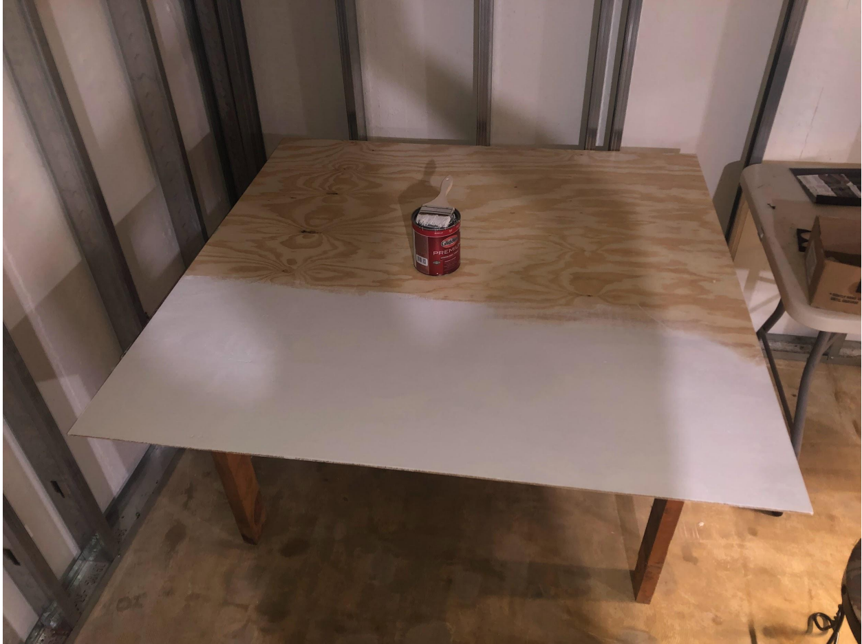
The sheet, with its best looking side facing up having its first coat applied
