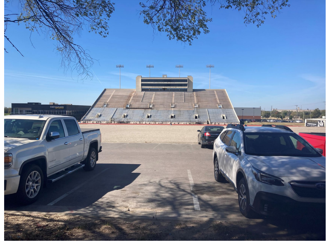
Concrete pillars for press box can be used to support the metal structure of tiered seating.
