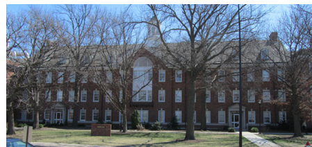
The new institute will be located in McKinley Hall
