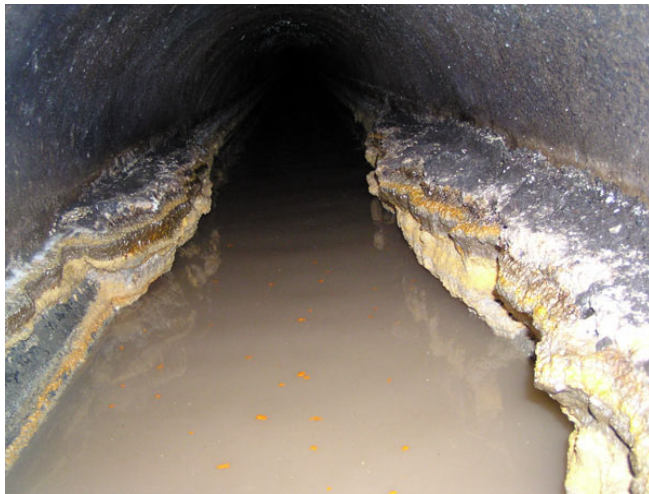
Grease can cause pipes to clog
