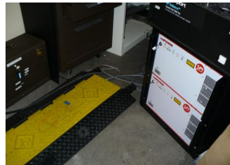
Figure 19: Wire Floor Bridge
