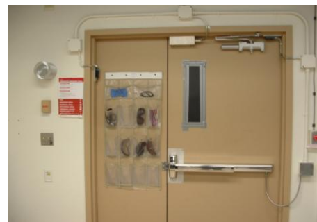
Figure 2: Eyewear Being Stored on Interior of Door
