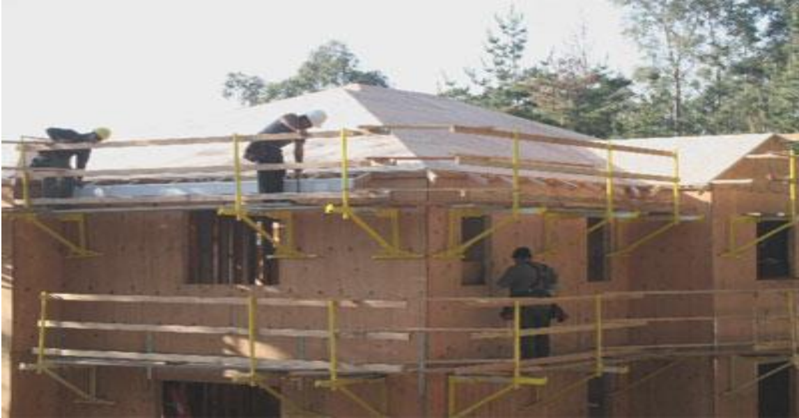
Figure 2.3: Carpenters bracket scaffold
