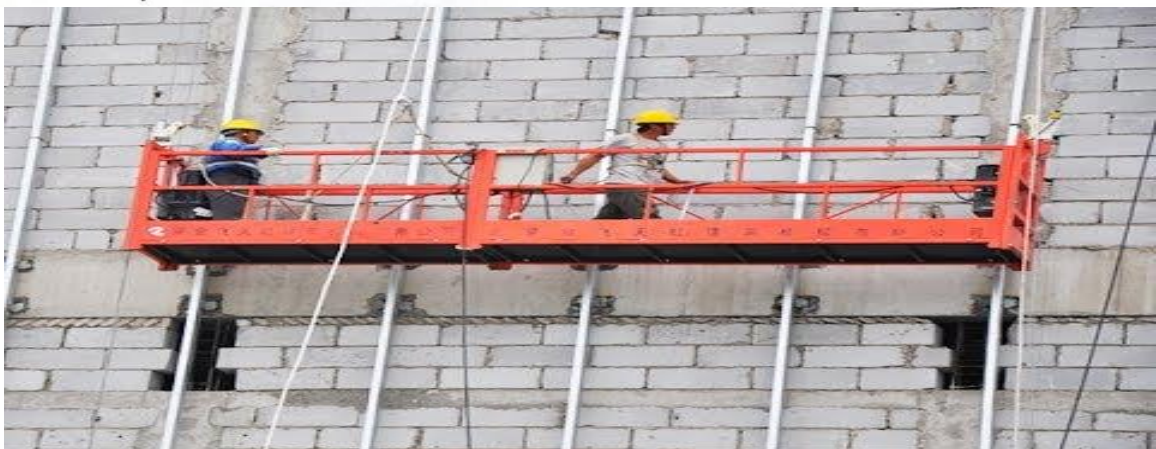
Figure 2.2: Suspension scaffold
