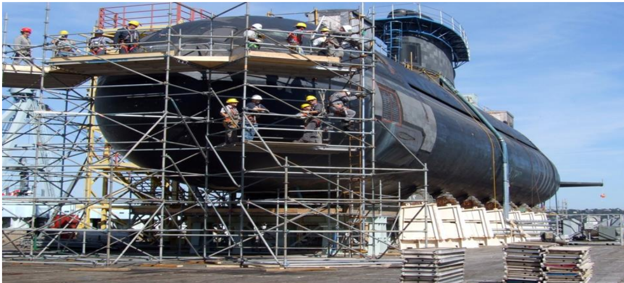
Figure 2.1: Self-supporting scaffold
