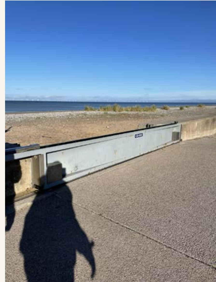
A community at risk of flooding
